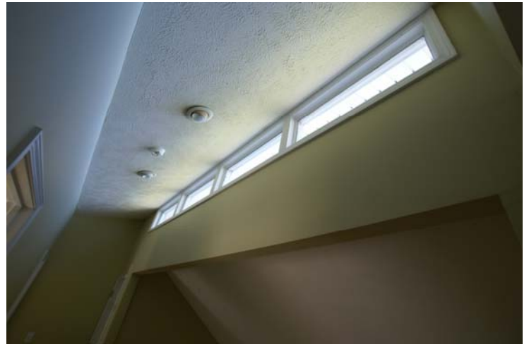
Upstairs Hall Roof Windows
